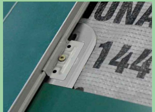
Above Sheathing Ventilation Spacer Shim
